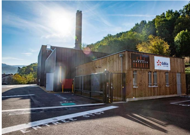
Local wood-fired boiler room supplying the Saint-Affrique urban heating network (Source : Causses Energia 2021)
