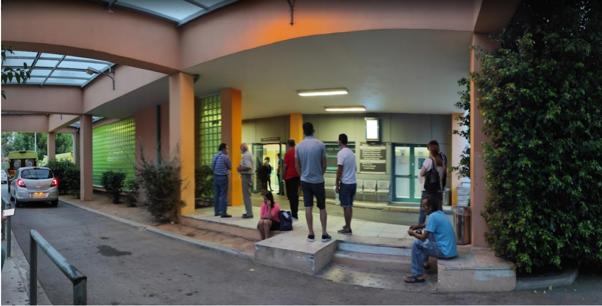
Entrance of the Emergency Department, NHOSP (Source: Valdimirios Poliakov, Google Earth, October 2020)
