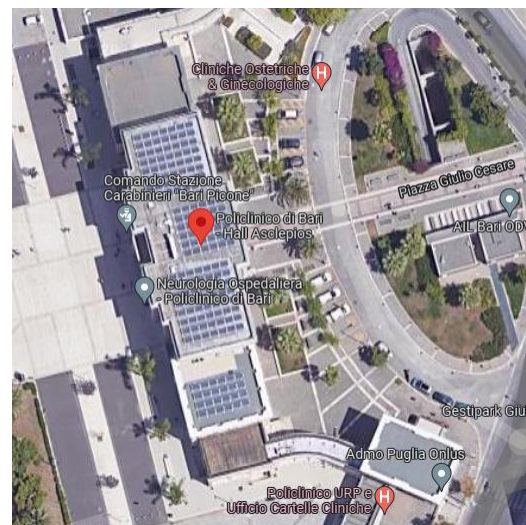
Photovoltaic panels on the roof of the Asclepios III building (Source: Google image, Maxar Technologies, 2022)
